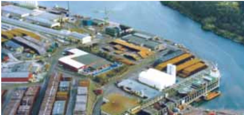
Coatings and linings for the Langeled Project were applied at Bredero Shaw's facility in Farsund, Norway
