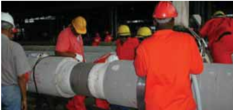
Advanced polypropylene joint protection systems for offshore pipelines
