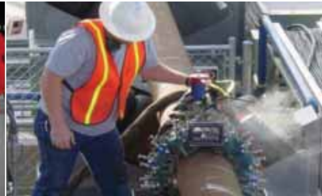
Automated high resolution pulse echo ultrasonic weld inspection
