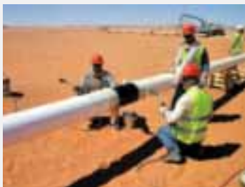
Canusa-CPS polypropylene sleeves being installed on a pipeline in Algeria
