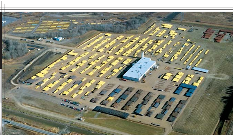
STACKS OF BARE PIPE AND PIPE COATED WITH YELLOW JACKET™ CORROSION COATING AT BREDERO - SHAW'S EXPANDED 34TH STREET FACILITY IN EDMONTON, ALBERTA.
